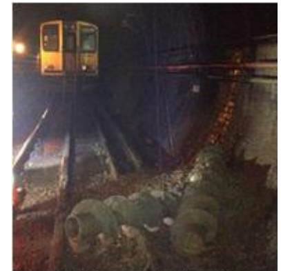
Rail staff spotted the drills which broke through into the tunnel
